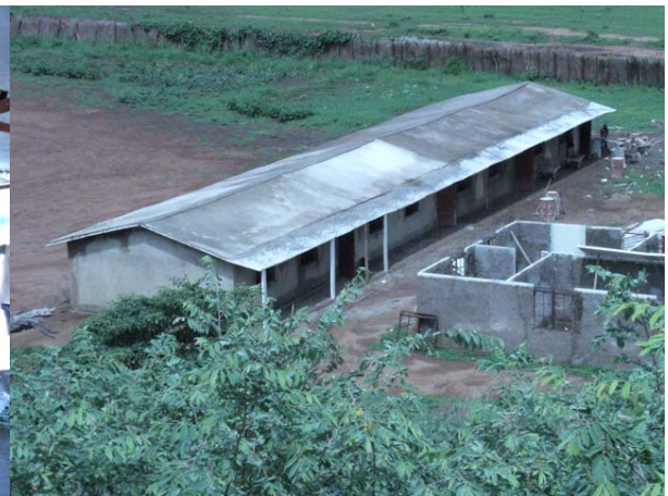
Complete view of first 4 classroom block near Completion
