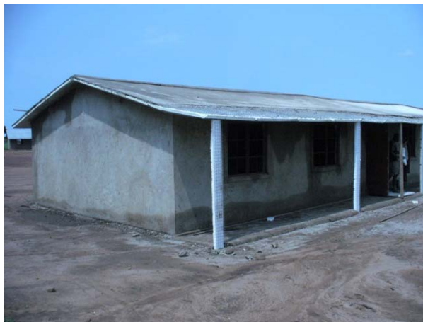
First 4 classroom block near completion.
