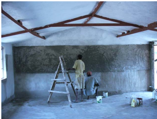
One classroom nearly finished.
