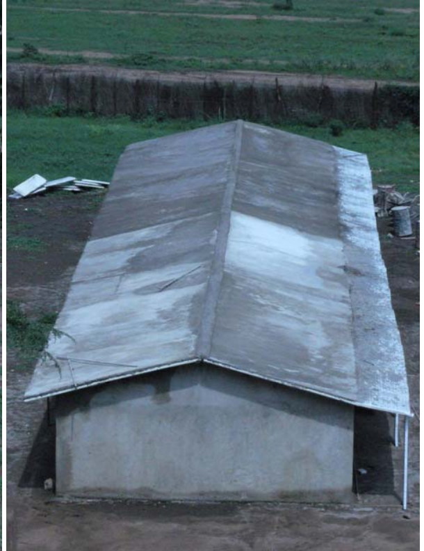
Nearly finished roof of first 4 classroom block.
