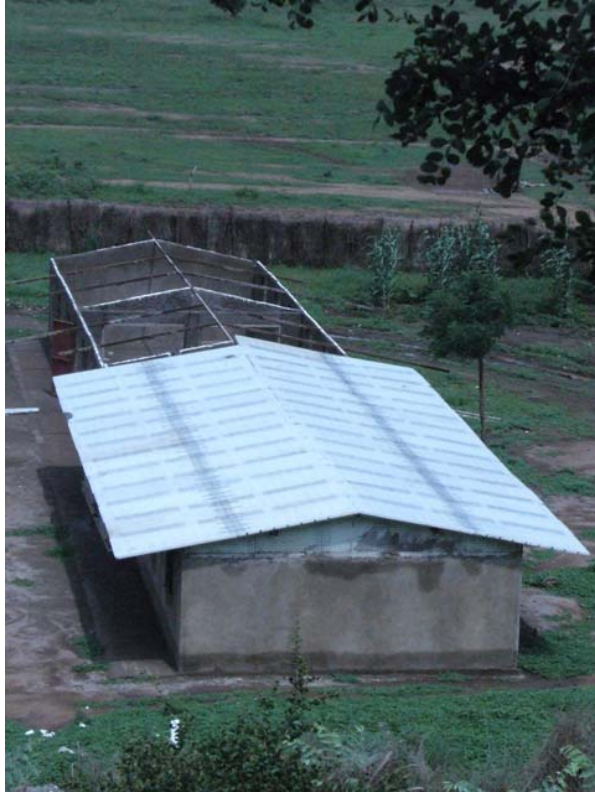
Second 4 classroom block still under roof finishing.
