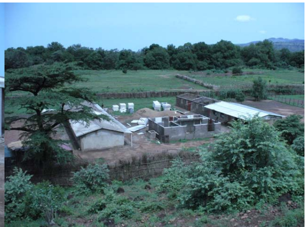
Whole view of the school construction.
