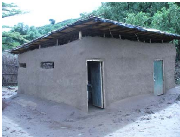
New temporary Kuron Health Care Centre which was commissioned for use 06/08/2007
