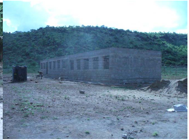
Permanent Kuron Primary Health Care Centre yet to be completed.
