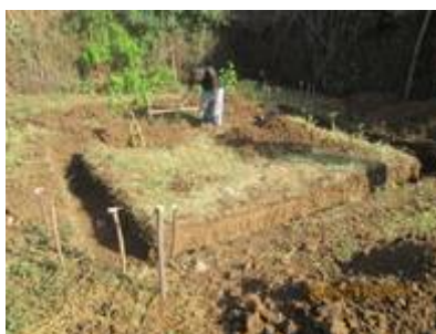
Ben Okeng making the foundation of Security House
